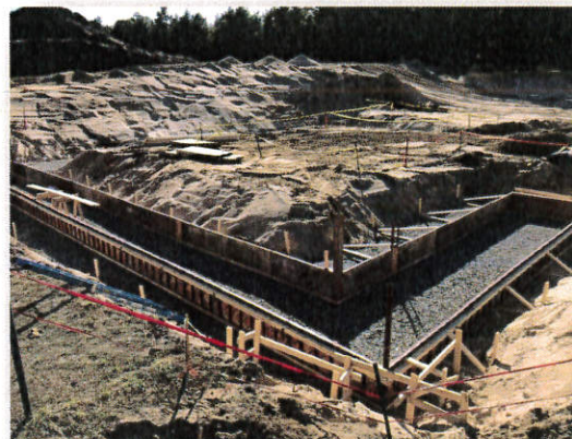
Picture of the Filtration Building Footprint
