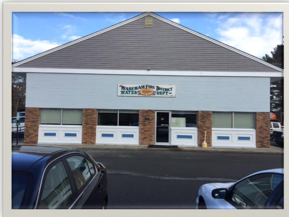
Picture 1: Refurbished Water Department Office after new roof and painting
