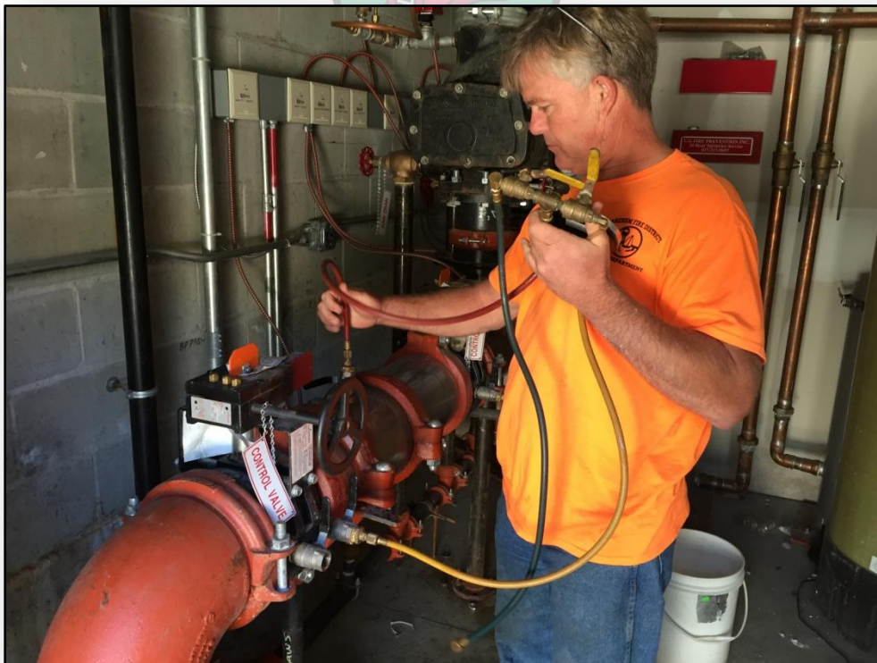
Picture 4: District Performing a Backflow Test
